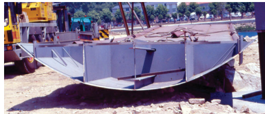
(b) Deck cross-section with circular segment shape.
